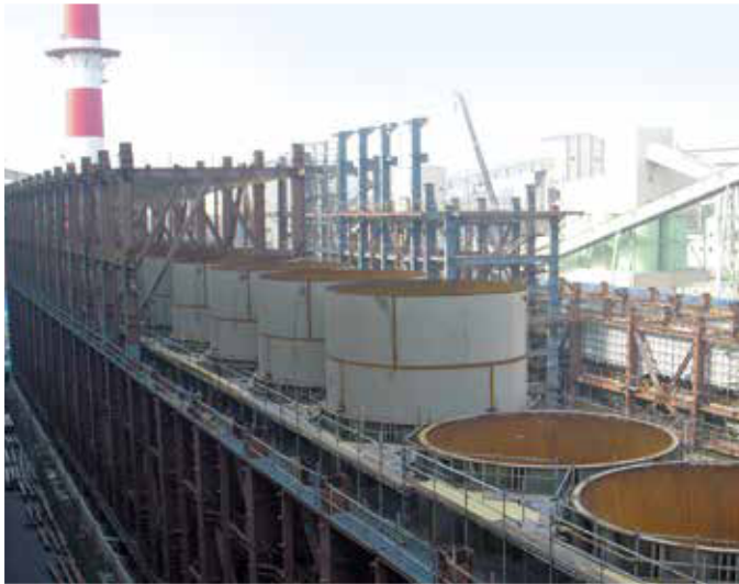
Proportioning bins under construction
